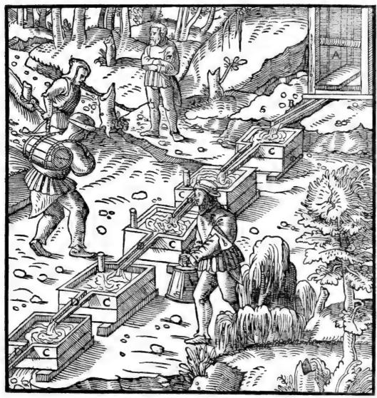
A-Mouth of the tunnel. B-Trough, C-Tanks. D-Little trough.
